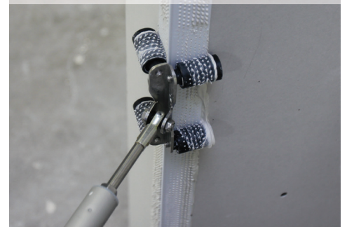
If using a compound tub apply mud/compound to drywall corner
