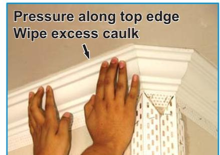
Step 3: You must apply a 1/2" bead of high quality white paintable adhesive caulk, such as Trim-Tex 700/710 caulk or Big Stretch from Sashco, along the front edge of the top flange of the Crown Molding. Apply 847 Spray Adhesive to the mud leg.
