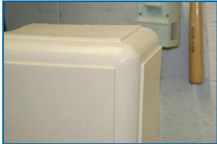
**Step 6:** Finish the installation by mudding, sanding and painting the bead as you normally would any other bead.
