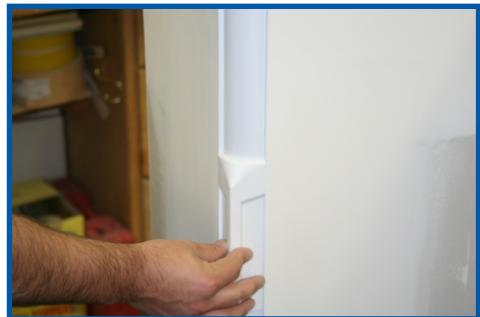
**Installation:** Cut Step A Bull adapter to the appropriate height to fit your baseboards. Install the adapter by applying 710 or 700 Adhesive Caulk or Liquid Nails onto the back of the adapter. Press the adapter into place and finish the installation by mudding, sanding and painting the adapter as you normally would any corner bead. The lower area of the adapter that will be covered with baseboard does not need to be mudded
