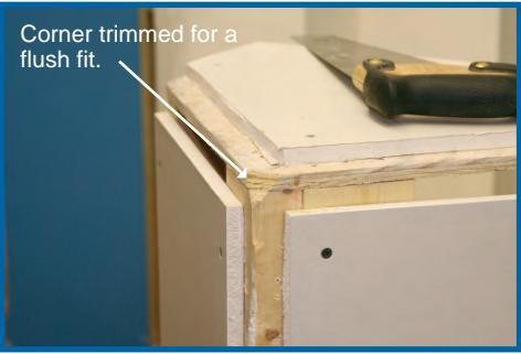
**Step 1:** When using  $\frac{1}{2}$ " drywall you will need to set the drywall back a  $\frac{1}{2}$ " for the  $\frac{3}{4}$ " Radius Step A Bull and a full 1" for the  $1\frac{1}{2}$ " Radius Step A Bull.
