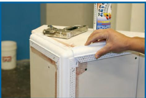
**Step 3:** Install the 3 way corner with  $\frac{1}{2}$ " divergent staples and Trim-Tex 847 Spray Adhesive.
