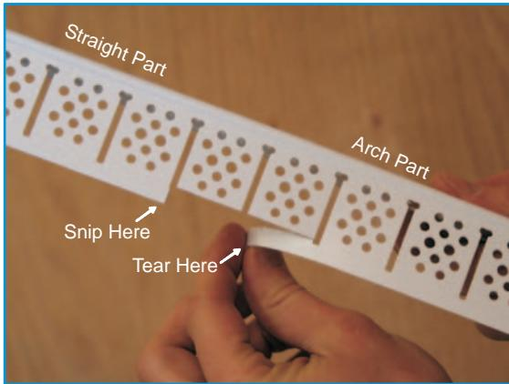
Snip the bead as shown above to leave part of the bead straight and the rest arched.
