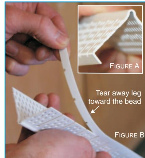
**Step 1:** Use minimal drywall setback on the Arch Plus 90° Combo Corner Bead. Make sure the edges of the board are cleanly cut. Ripped or rolling paper will prevent the mud legs of the bead from sitting flat on the wall. Do not use the tapered edge of the board for outside corners.
