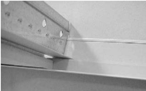
Correct shadow molding installation
