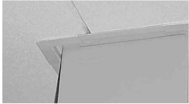
**Option A:** Shadow Molding is the most user-friendly; items #7875 or #7897 (seismic) are recommended.
