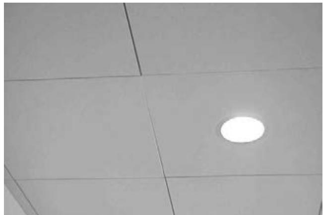
These are usually panels that receive sprinkler heads and high hat fixtures. **The holes for penetrations must be large enough to allow the panel to be properly aligned.**
