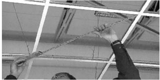
Do not attempt to install Vector panels until the suspension system is properly squared.
