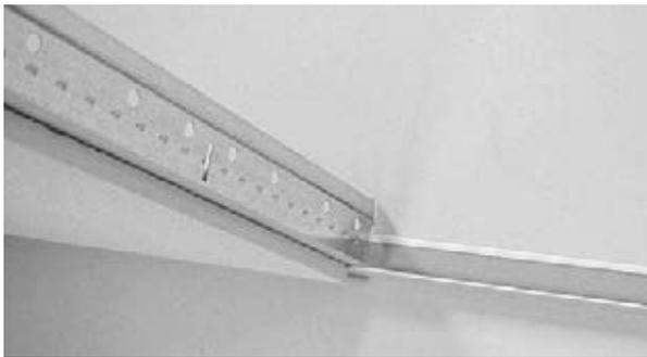
Correct "L" wall molding installation with suspension resting on molding.
