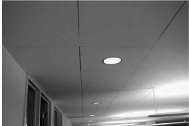
Unlike in this example, Vector panels should maintain a 1/4" reveal between panels in all directions.
