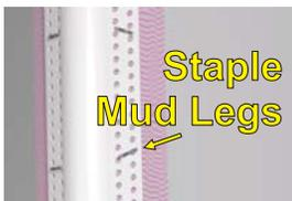
**Step 4:** Staple the mud legs every 6" with 1/2" staples. Reapply pressure to the mud legs as needed to guarantee a proper bond. On arched beads you may need to staple every tab. Securely attaching the bead minimizes the chance of edge cracking. DO NOT install the bead with nails or drywall screws.
