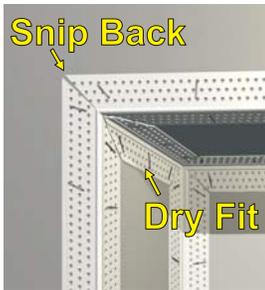
**Step 2:** On vertical corners, do not allow the bead or bulladapter to touch the floor. Always install with a 1/2" gap to prevent structural settling from cracking the mud. If you're using 2 ways, 3 ways or Bulladapters install these first with 847 Spray Adhesive & Staples. To glue the bead to the molded corners, put a dab of Bondaflex 700 Caulk on the tabs of the corners. Where beads meet, snip back mud legs as shown. Do not overlap mud legs. Dry fit as needed.
