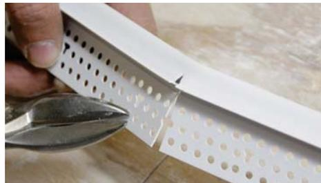
Next, flip the bead over and snip the mud leg all the way through the mud bump and into the back of the gasket.
