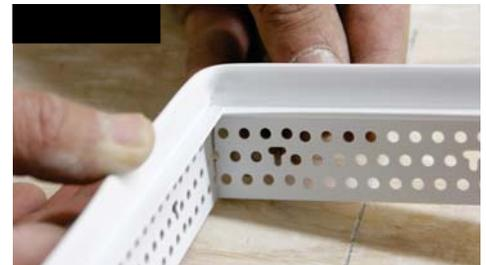
Make sure the front of the gasket is not snipped and bend the bead to ensure it forms a nice clean inside corner.
