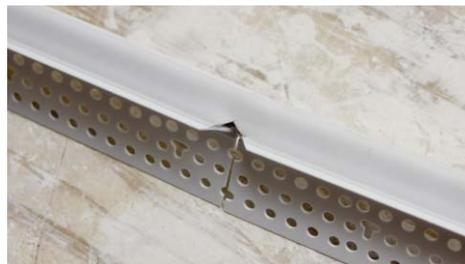
Next, flip the bead over and notch out the "V" slightly going into the gasket.
